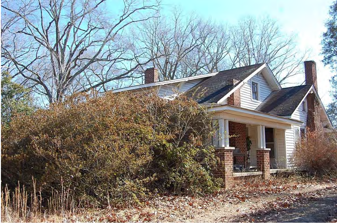
William T. and Doris W. Redwine Farm, House, Façade (Overgrown) and Side (West) Elevation, Looking South.
