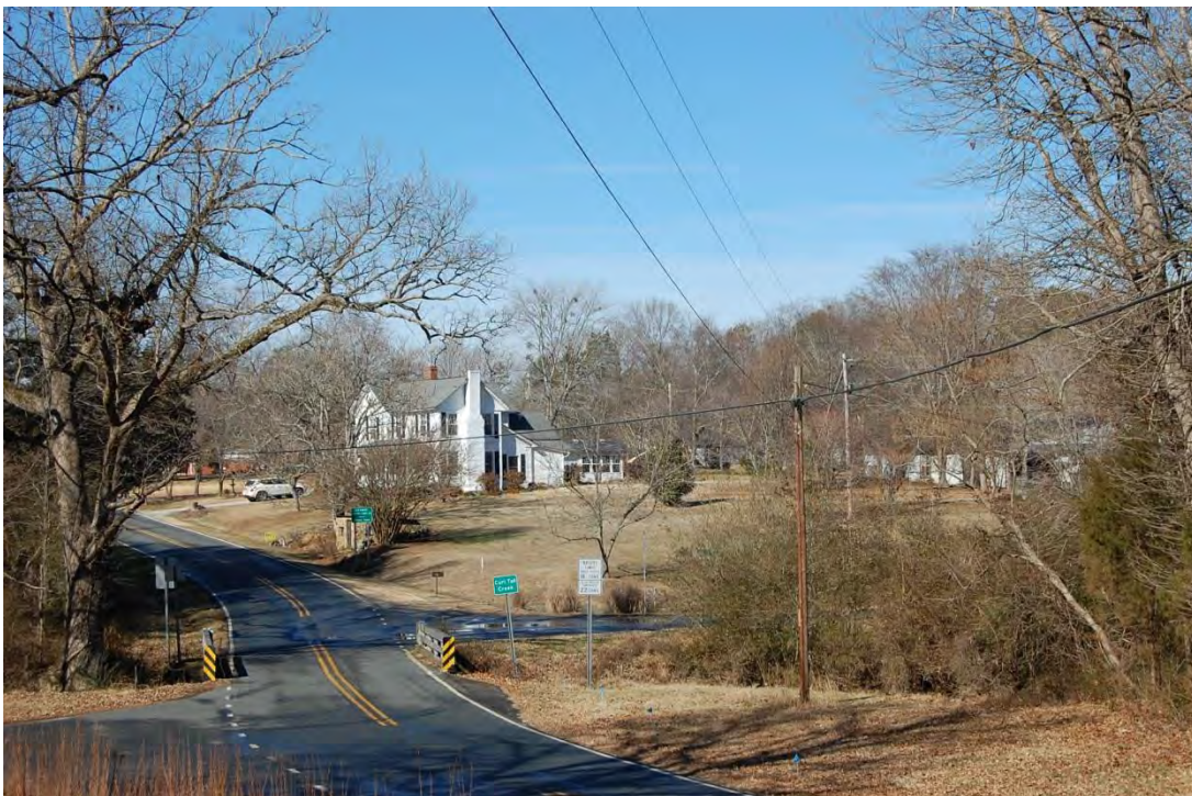
J. Henry and Amelia Arey House, Overall View, Looking Northwest Along Gold Branch Road.
