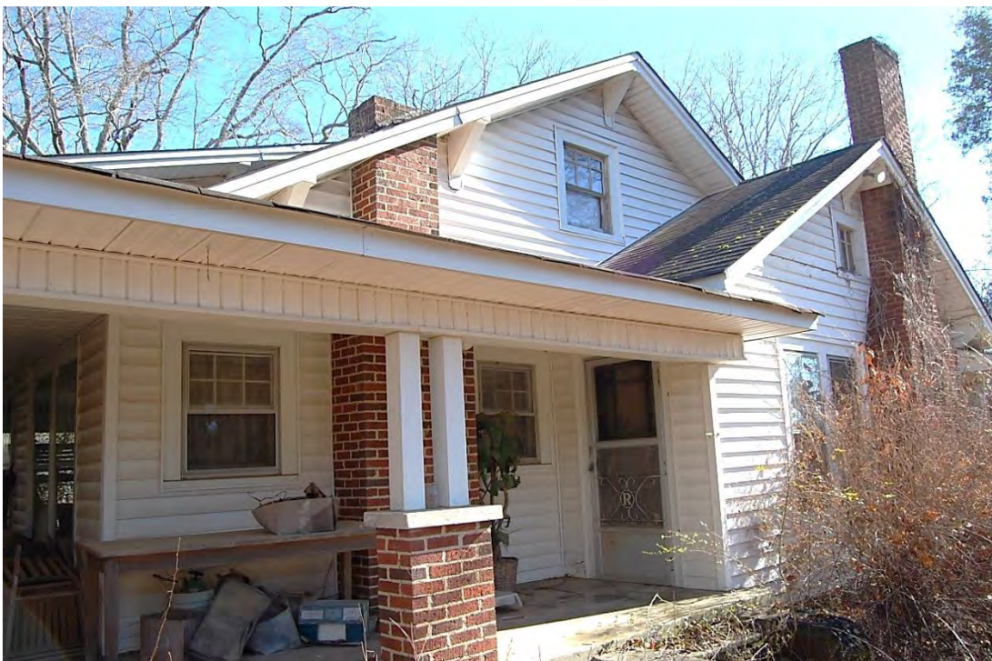
William T. and Doris W. Redwine Farm, House, Side (West) Elevation, Looking South.
