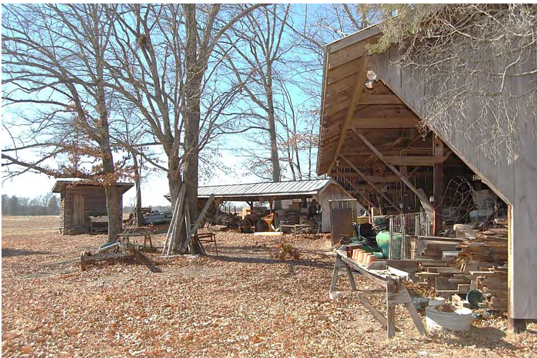
William T. and Doris W. Redwine Farm, Modern Equipment Sheds, Looking West.
