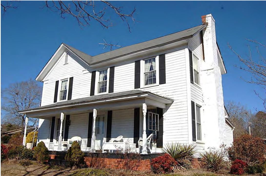
J. Henry and Amelia Arey House, Façade (West Elevation), Looking Northeast.
