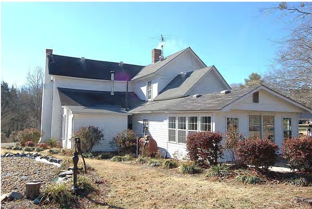
J. Henry and Amelia Arey House, Rear (East) Elevation, Rear Wing, Rear Shed, Rear Ell, Modern Sunroom, Enclosed Rear Ell Porch, and Shed Addition, Looking West.
