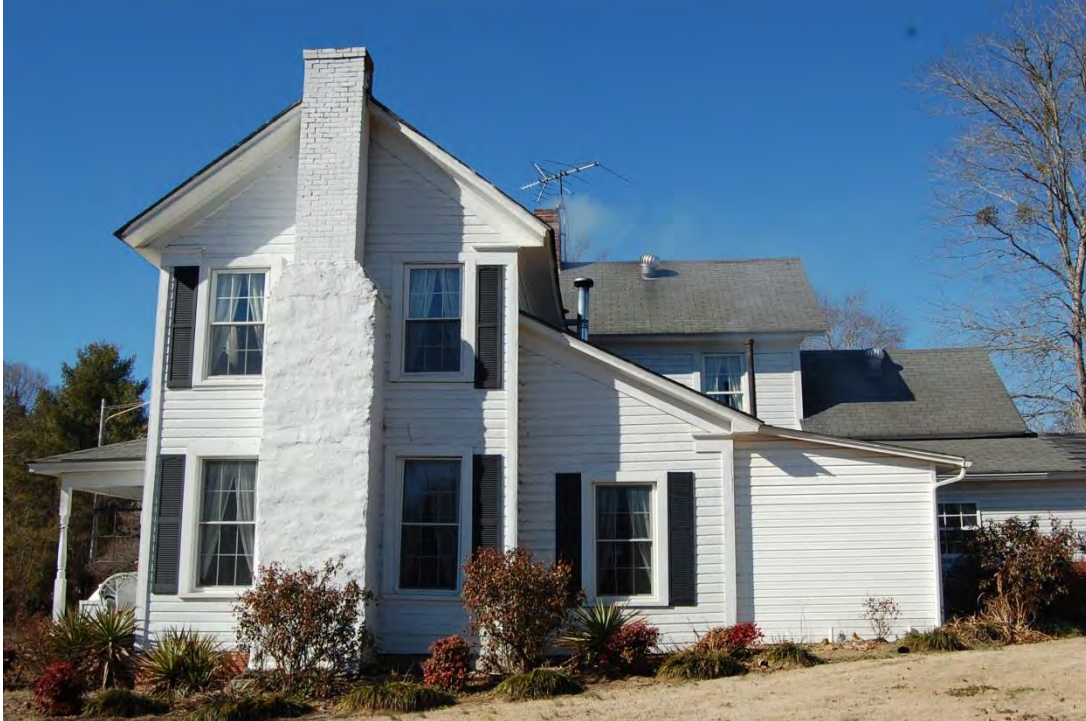
J. Henry and Amelia Arey House, Side (South) Elevation, Rear Shed and Addition, Looking North.
