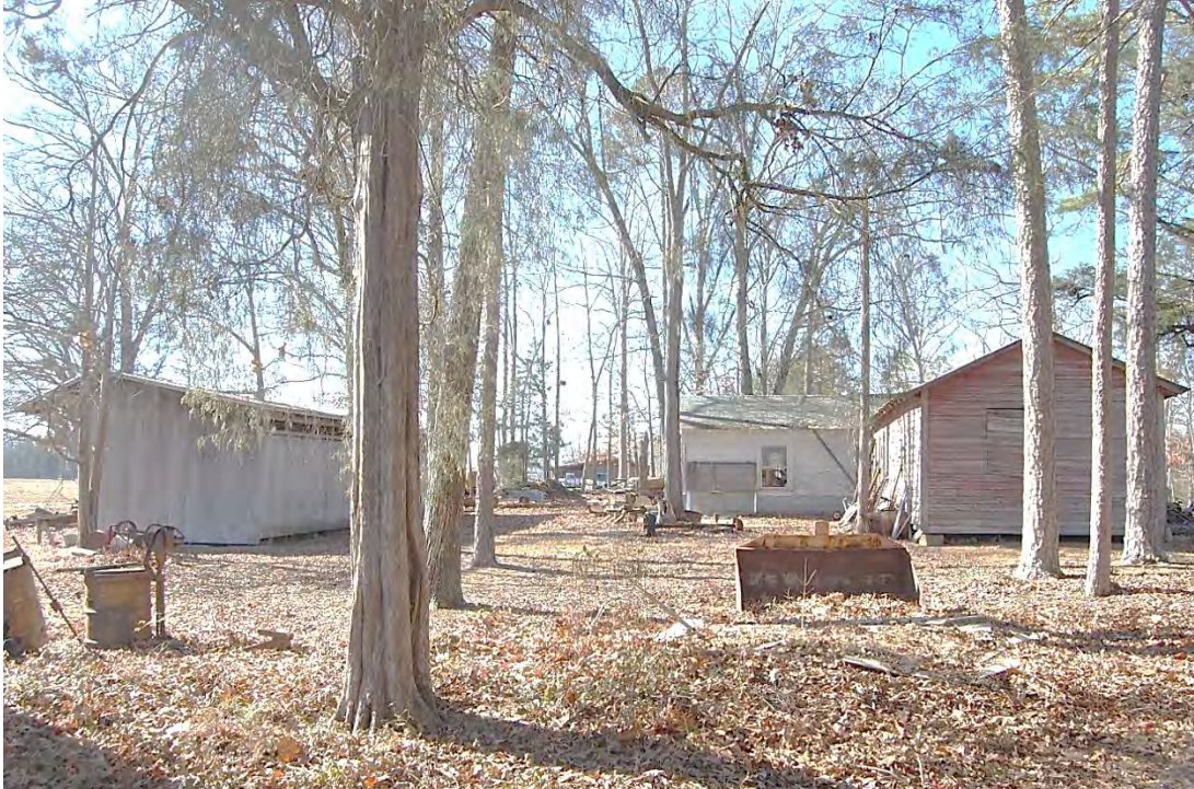
William T. and Doris W. Redwine Farm, Modern Equipment Sheds (Left and Background) and Original Equipment Shed (Right), Looking West.
